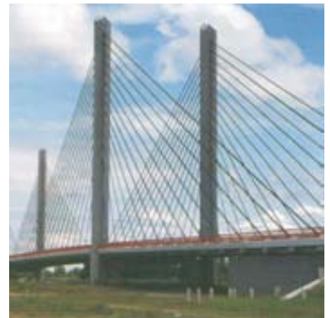
Papaloapan Bridge La Tinaja- Cosoleacaque Highway
