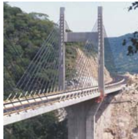
Quetzalapa Bridge Mexico-Acapulco Highway
