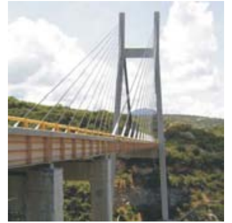
Barranca El Cañon Bridge Mexico-Acapulco Highway
