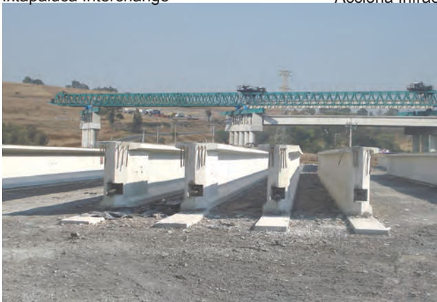
Ooapas Bridge, Morelia-Maravatío Highway
