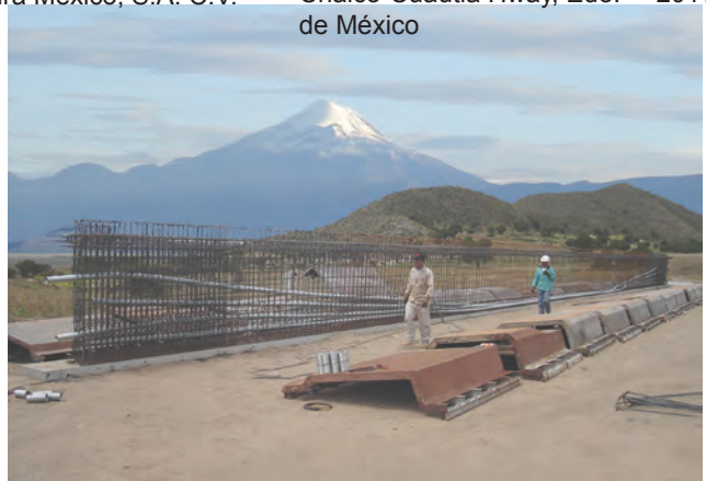
Arroyo Bridge, Amozoc-Perote Highway
