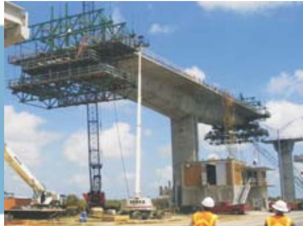
GIWW Bridge, Texas, USA
