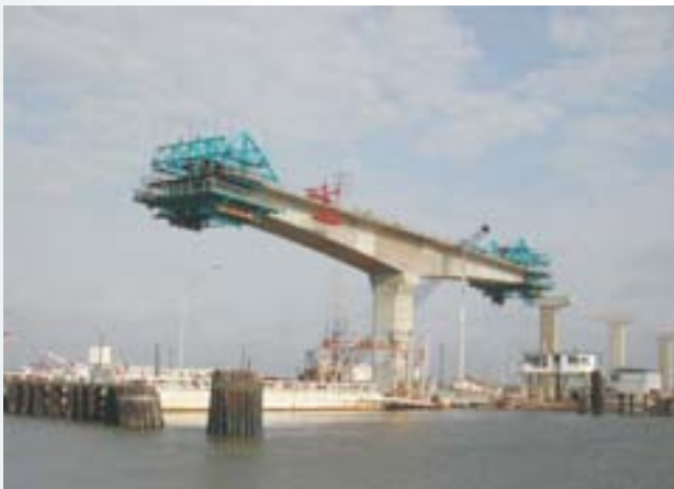
Quintana Bridge, Texas, USA
