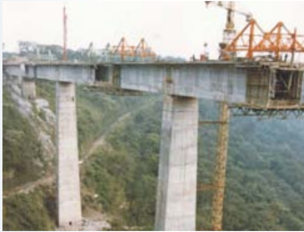
Metlac Bridge, Mexico
